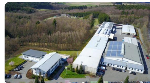
An aerial photo of our premises in Ingelbach-Bahnhof
